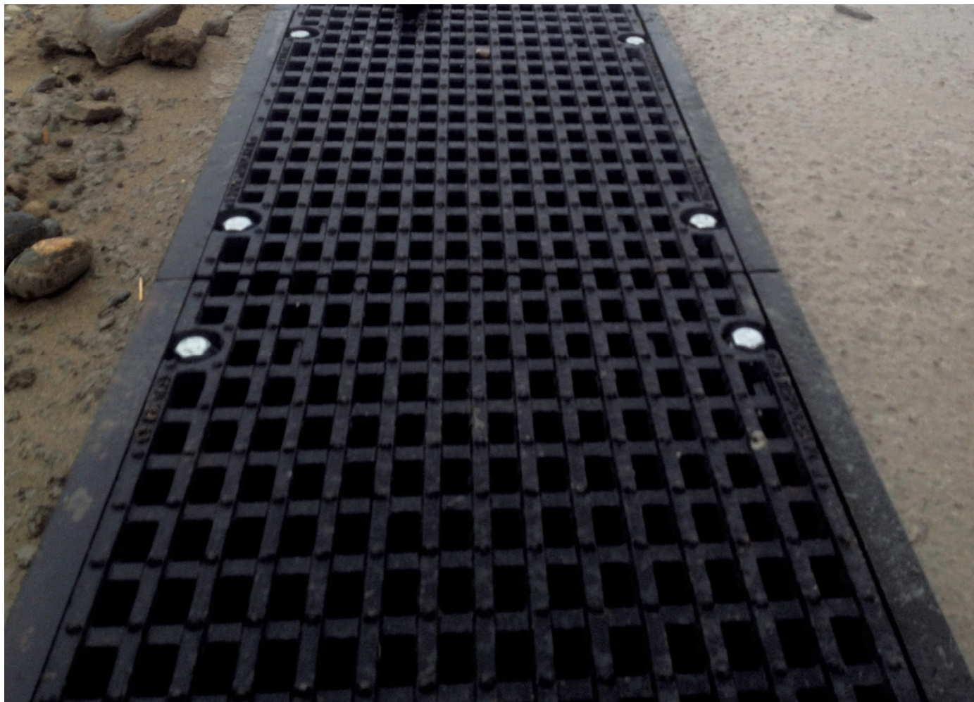
Krasnodarsky Krai, Derways plant, drainage gutters BGZ-S with cast-iron grates
