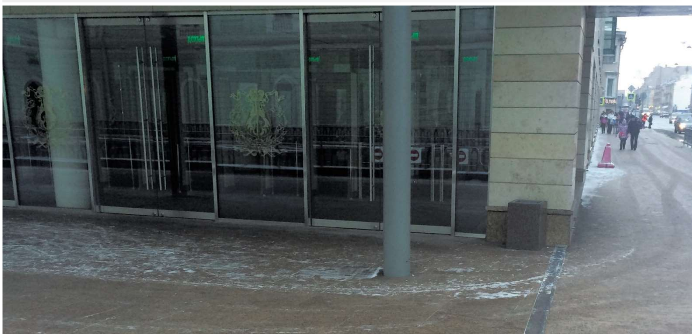
Saint Petersburg, the Mariinsky Theatre, drainage gutters Hidrolica® Standart with galvanized grates
