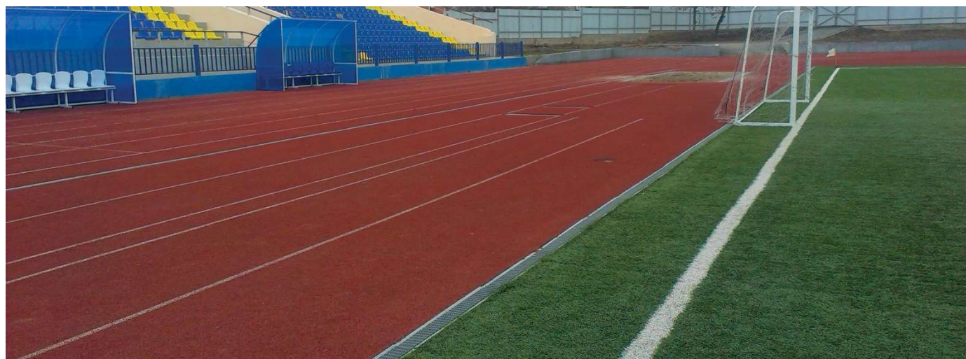
Stadium in Novoshakhtinsk, drainage gutters Gidrolica® Standart Plus with galvanized steel grates
